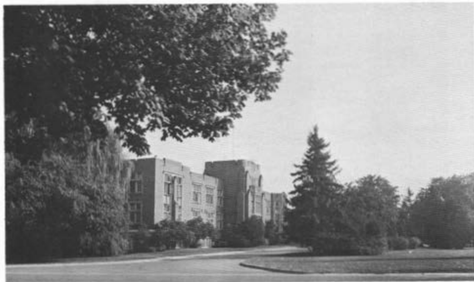
The William Saunders Building at the Central Experimental Farm, which houses the vascular plant botanists and mycologists and their associated herbaria.
