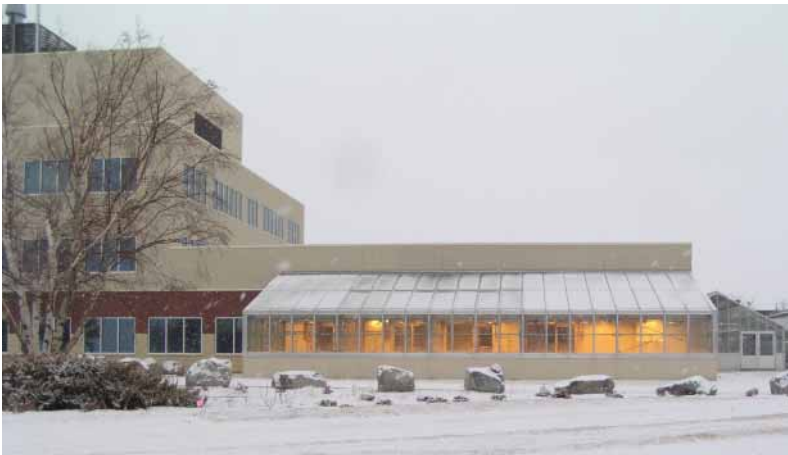
The insect containment facility greenhouse at the Lethbridge Research Centre, Agriculture and Agri-Food Canada, Lethbridge, Alberta.
