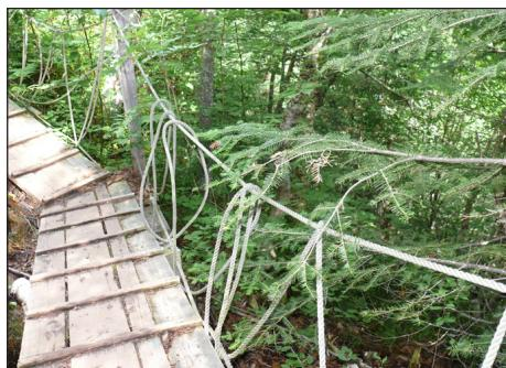
Figure 20. Insecure bridge over a stream on a hiking trail.
